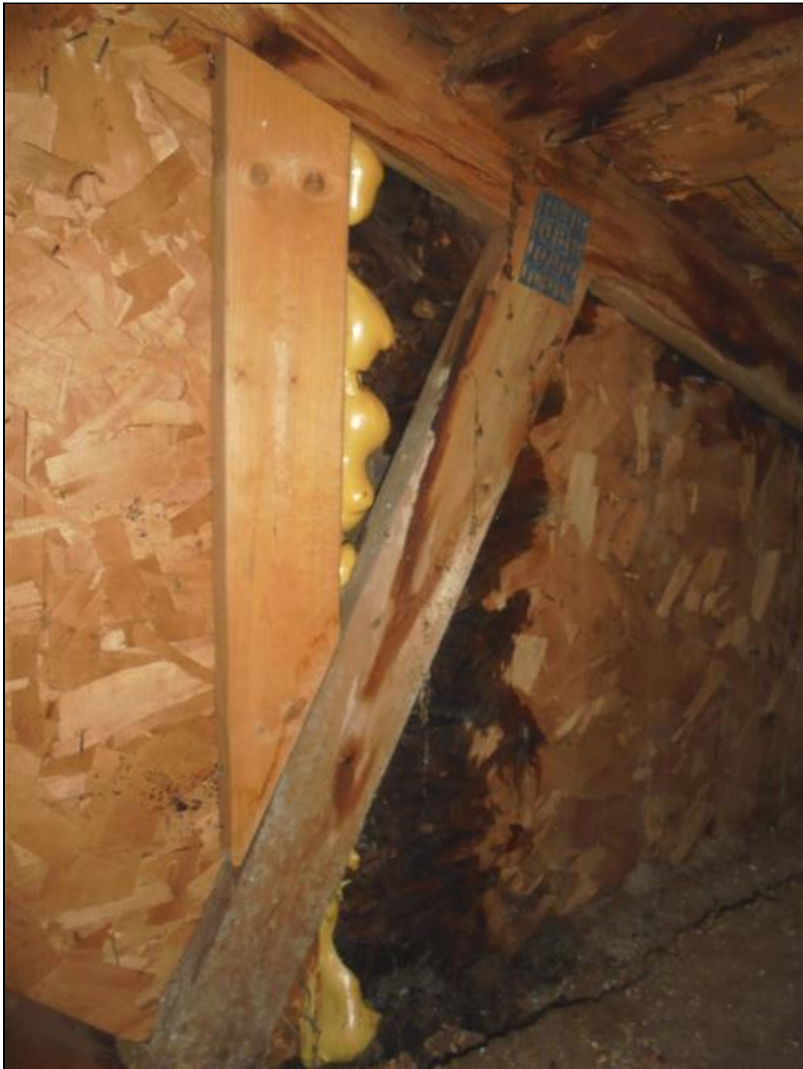
1.5 Item 1(Picture) Water damage in attic above family room
