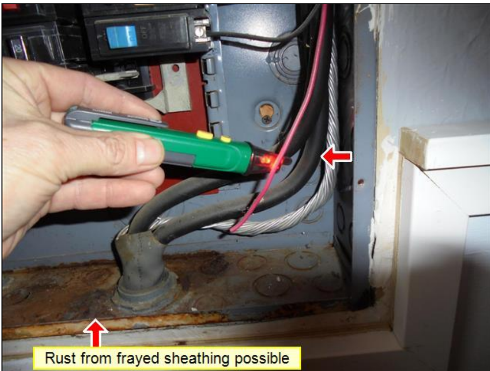
9.1 Item 3(Picture) Hot wire hanging free in box and rust
