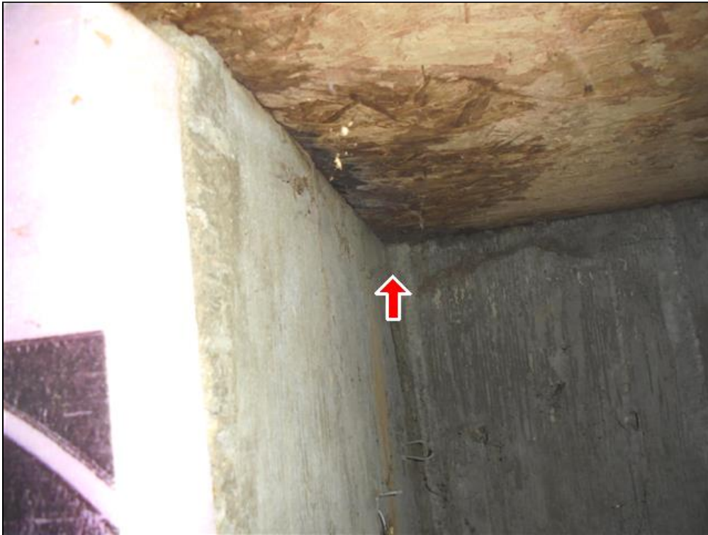
7.0 Item 4(Picture) Moisture intrusion under chimney in crawlspace.
