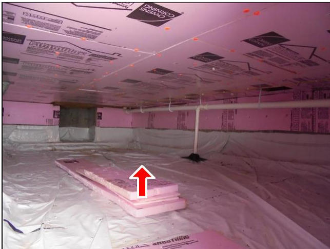
7.0 Item 3(Picture) Area of vapor barrier where water is pooling under barrier
