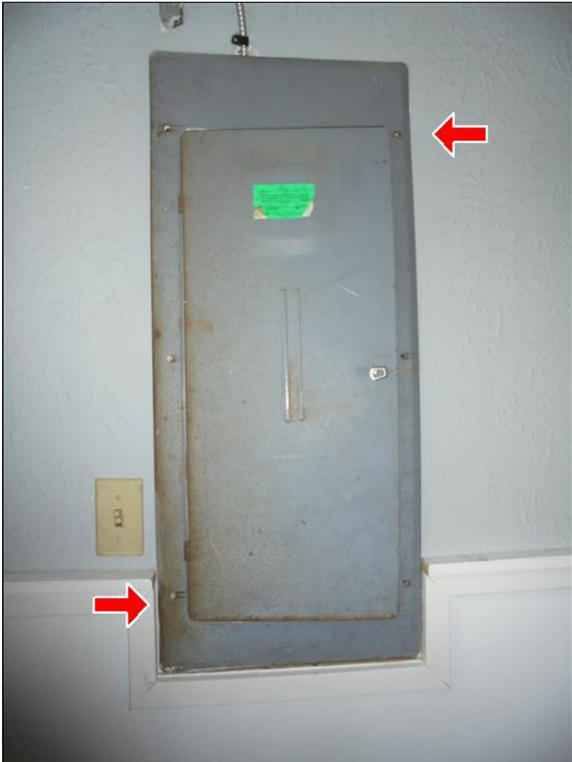
9.1 Item 1(Picture) Only 2 screws securing box cover
