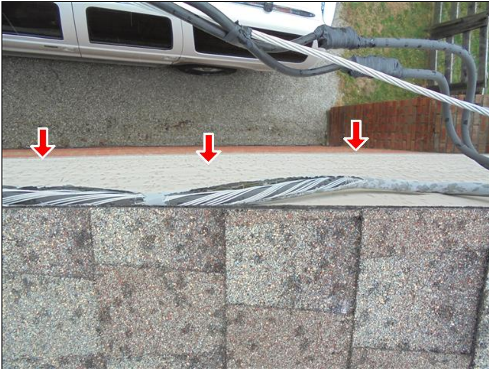
9.0 Item 2(Picture) Split wire sheathing
