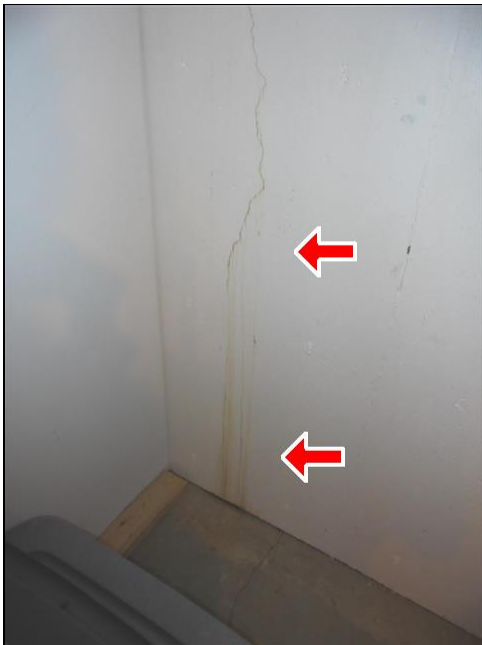
7.0 Item 1(Picture) Water staining wall
