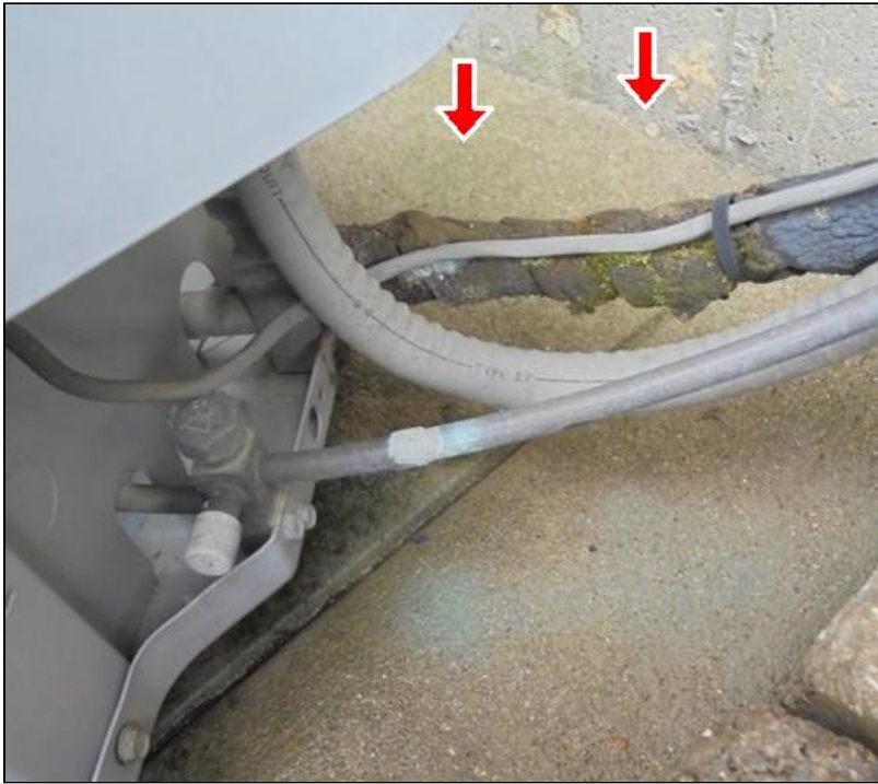
10.8 Item 2(Picture) Damaged foam sleeve
