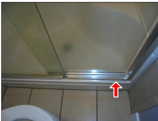
6.5 Item 2(Picture) Shower door in the closed position
