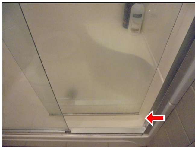
6.5 Item 1(Picture) Bottom of shower door not on track
