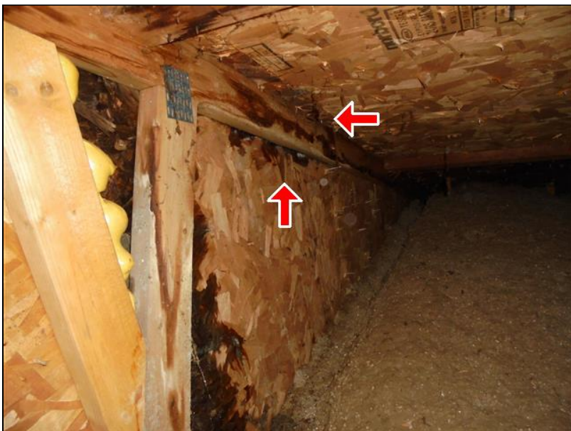
1.5 Item 3(Picture) Moisture traveling down joist
