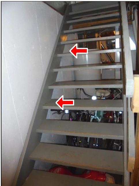
5.3 Item 1(Picture) Basement steps loose, not secured to wall
