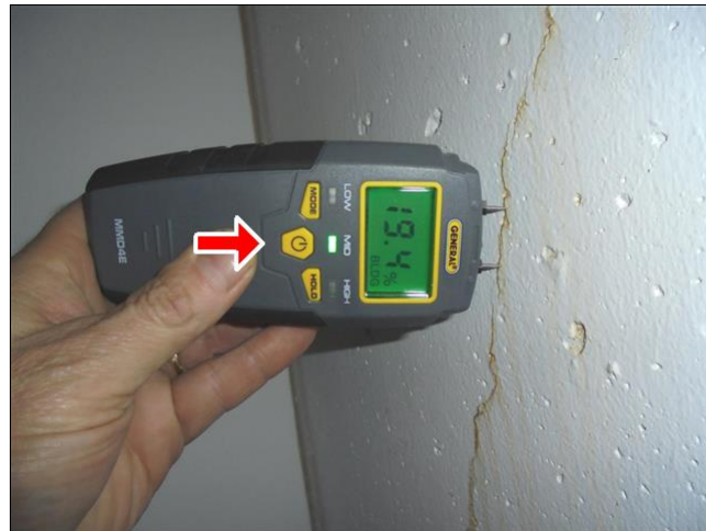
7.0 Item 2(Picture) Moisture meter showing medium moisture in the area
