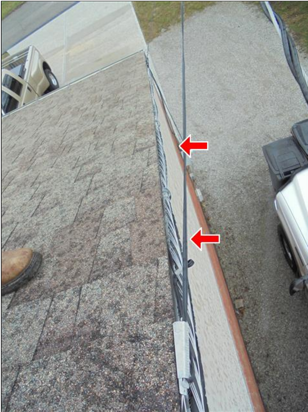
9.0 Item 1(Picture) Wire sheathing split going down side of house
