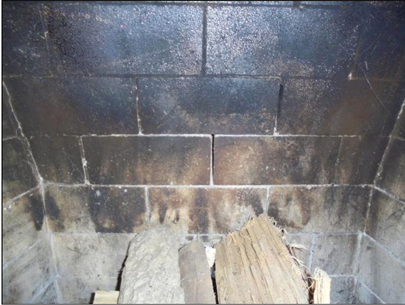
10.5 Item 1(Picture) Missing mortar
