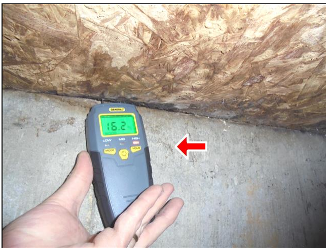
7.0 Item 5(Picture) 16.2 High level of moisture at chimney base
