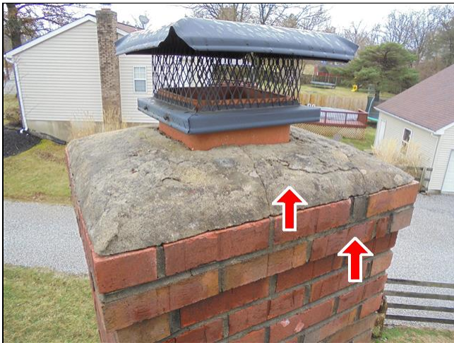
1.2 Item 1(Picture) Chimney crown
