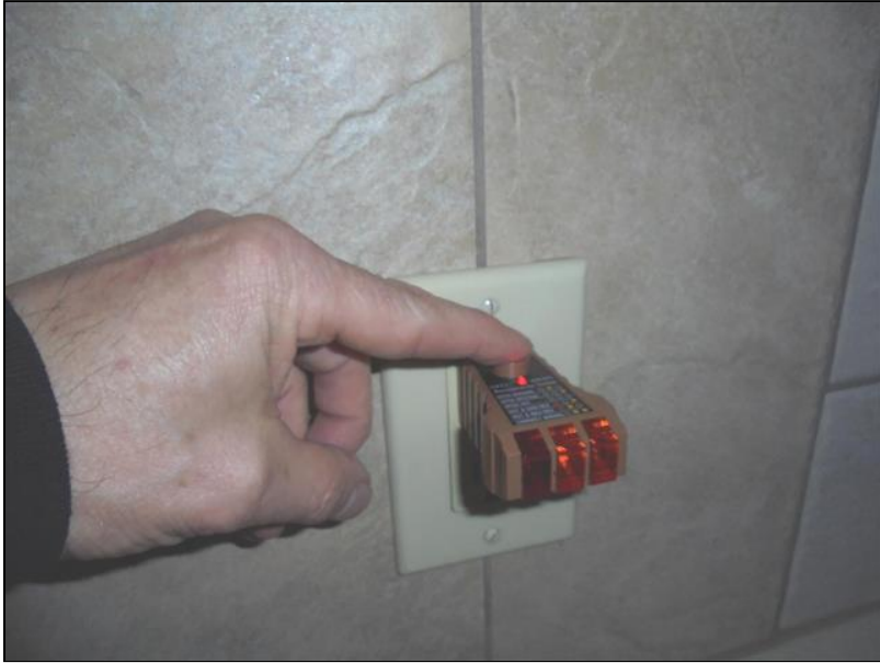
4.8 Item 1(Picture) GFCI not working Kitchen
