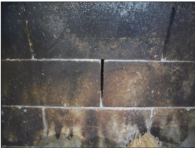
10.5 Item 2(Picture) Close-up of missing mortar
