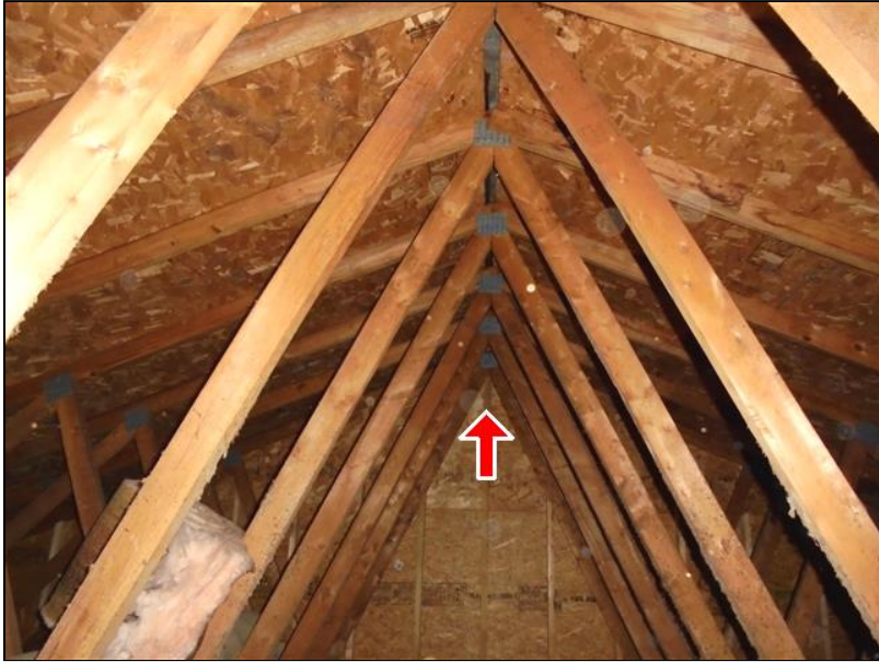
1.5 Item 4(Picture) Daylight showing in attic
