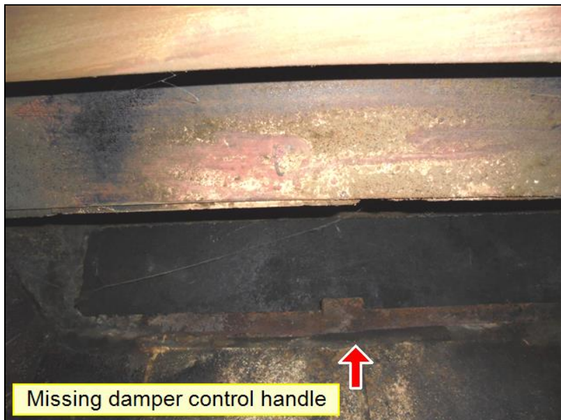
10.7 Item 1(Picture) Missing damper arm
