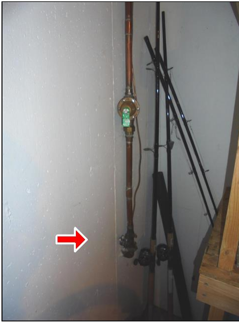
8.3 Item 1(Picture) Main water shut off
