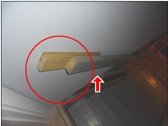
5.3 Item 2(Picture) Improper handrail
