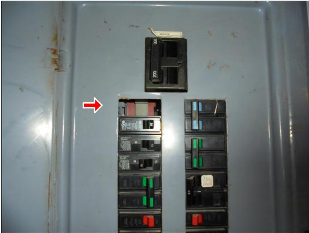
9.1 Item 2(Picture) Missing knockout cover
