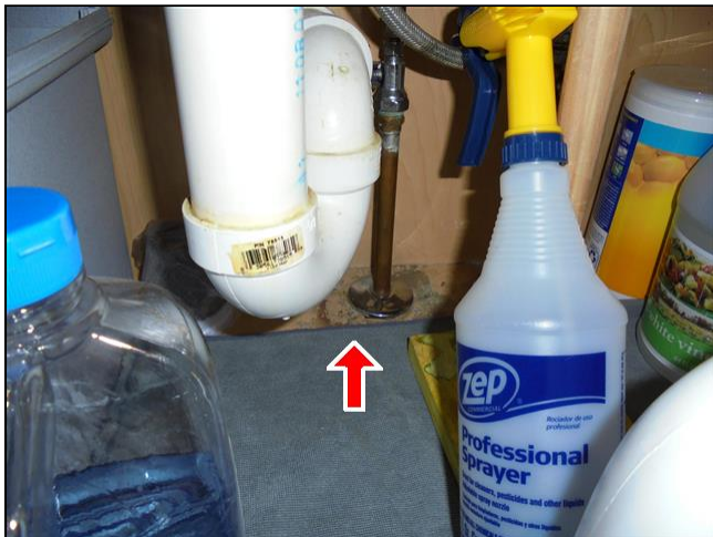
4.5 Item 1(Picture) Prior water damage under sink
